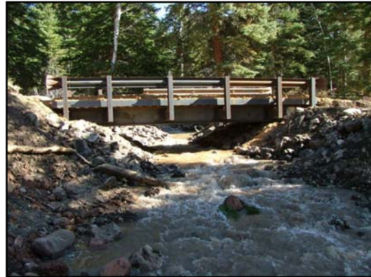
Figure 3: A new bridge, which has replaced a previously existing culvert that was considered a partial fish migration barrier.
