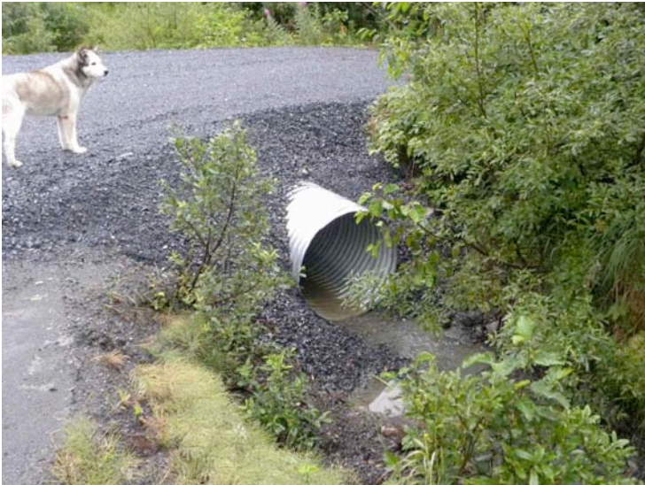
Figure 13: Looking upstream at the downstream side of the Bartley driveway culvert. This ditch now drains stormwater from the City Baler.
