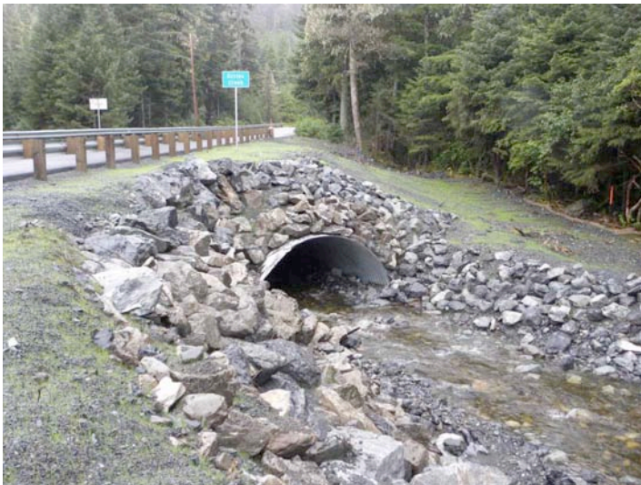
Figure 2: Looking upstream at the outlet of the new Eccles Creek culvert.
