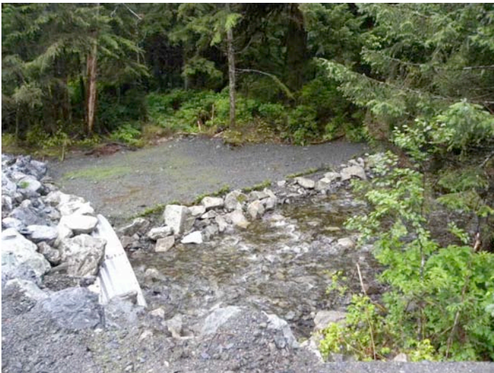
Figure 7: Looking east at the upstream side of the Eccles Creek culvert.
