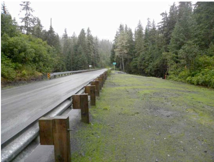
Figure 1: Looking south at Eccles Creek / Whited Road.
