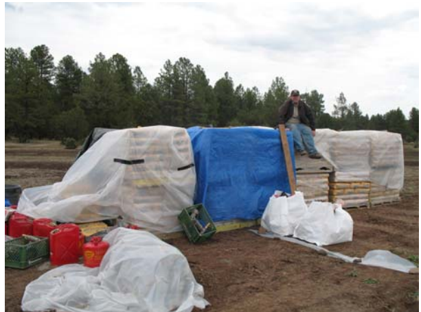
87,000 lbs of concrete
