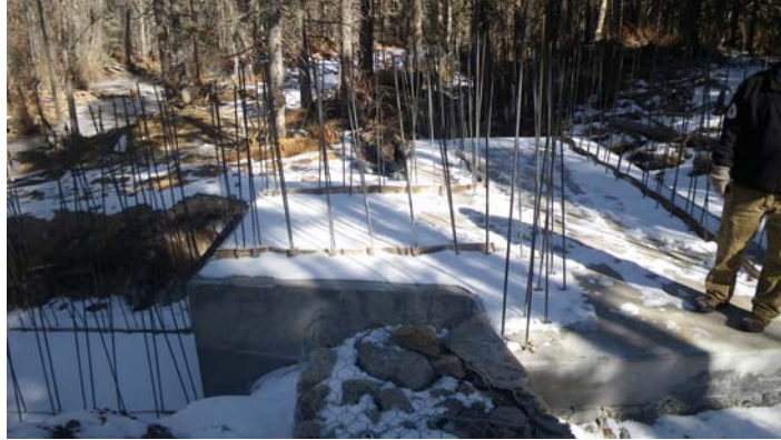
Barrier re-construction on Alamitos Creek, NM
