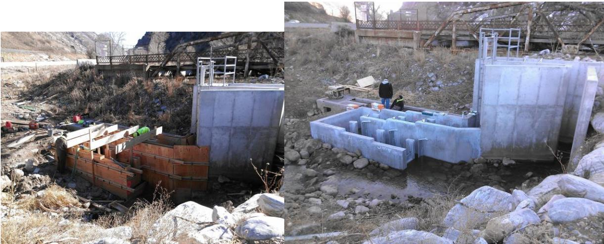
*New fish ladder at the Mouth of Weber Canyon. During 2013 over 1100 fish of all species moved through this fishway around the diversion dam. Biologists observed a high velocity bottleneck in the fishway at high flows, when fish typically move the most. The final concept was a fish ladder that is active only at high flows, which enters back into the top of existing fishway.*
