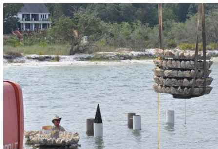
Ecodisc Breakwater Installation, Pensacola Bay, Florida. Photo Credit: Heather Reed.
