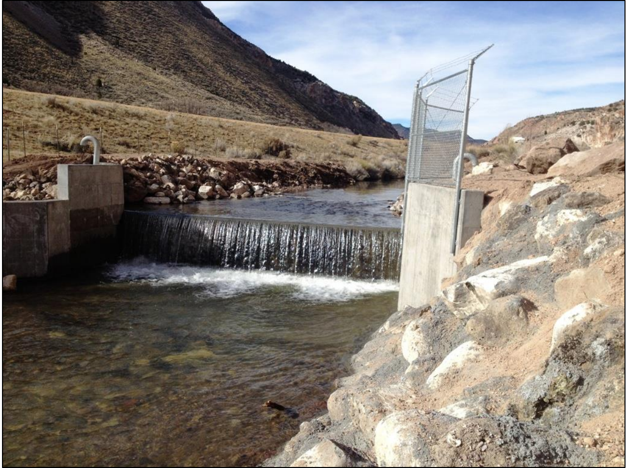
Figure 2. Clear Creek fish passage barrier.
