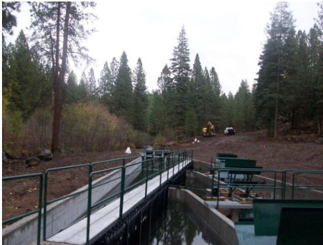
Paddlewheel cleaning mechanisms (left) and the completed fish passage channel (right; photo courtesy of Cascade Stream Solutions)
