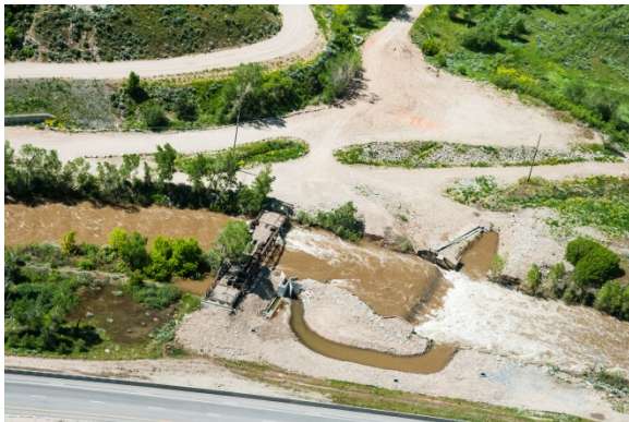
The lower Weber River Diversion after initial construction in 2011.
