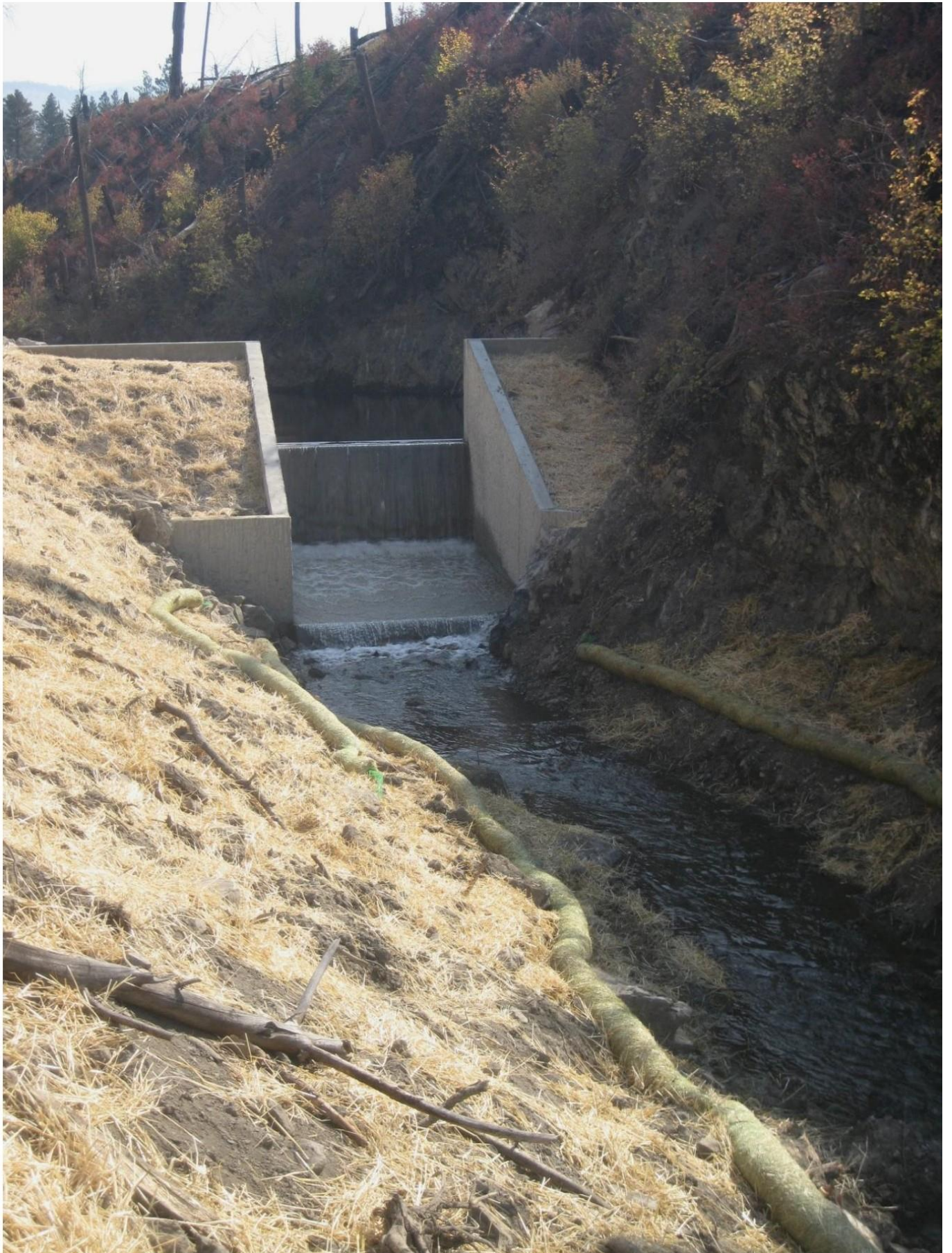
Figure 5. Completed Elkhorn Creek fish barrier September, 2012.
