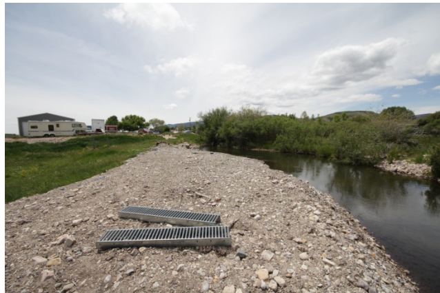
Photo 2: Bank Stabilization Area.
