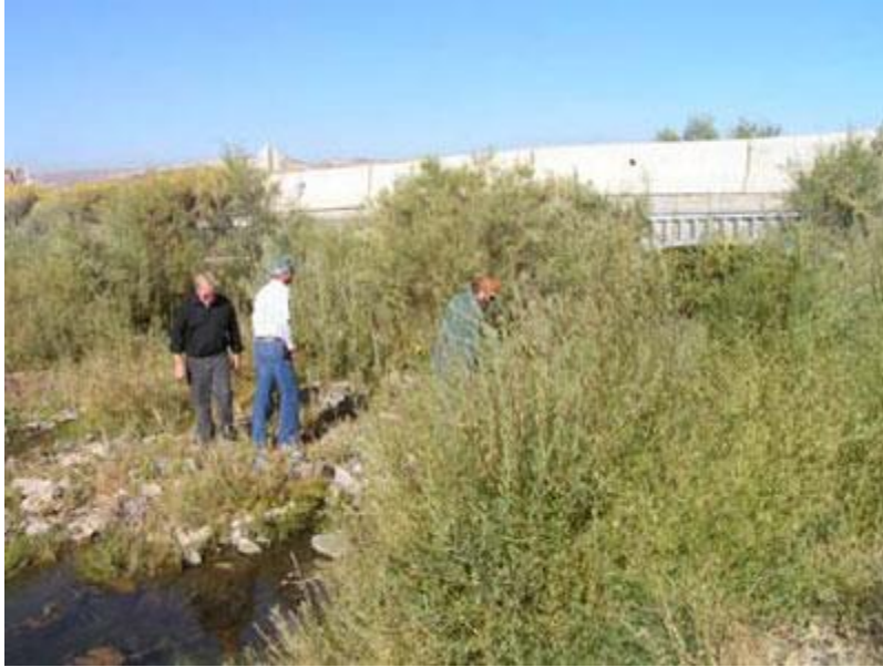
Figure 3. Bridge culverts under road to Newmont Mining Corporation's Cooling Towers.
