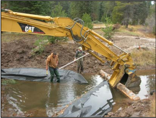
Forest Service crews install channel grade control and bank stabilization structure.
