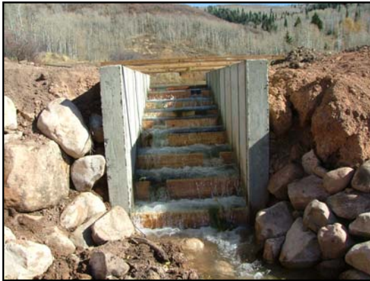
Figure 2: New fish ladders constructed on both ponds with wooden steps in place.
