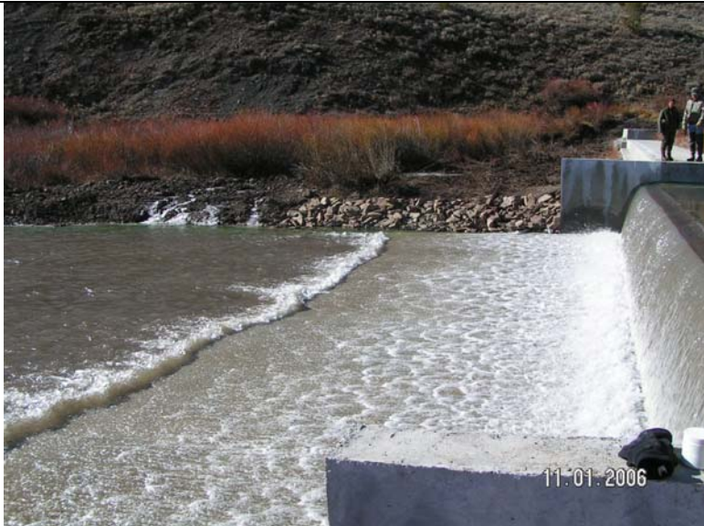
After completion of phase 1. Photo taken November 2006.
