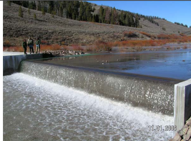
After completion of phase 1. Photo taken November 2006.
