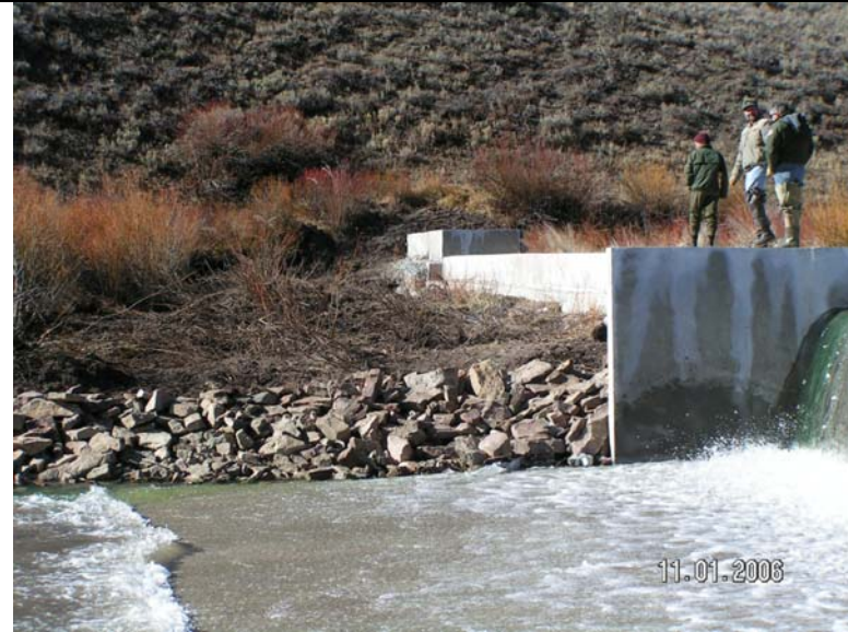
After completion of phase 1. Photo taken November 2006.
