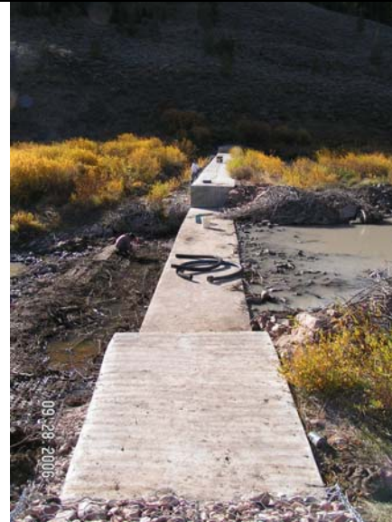
Start of construction, side view. Photo taken September 2006.
